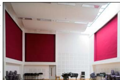
The fabric is attached to the slats by Velcro. The male half of the Velcro is secured along the edges of the slats, while the female half is sewn horizontally onto the back of the fabric – an intricate process done painstakingly by hand at J&C
